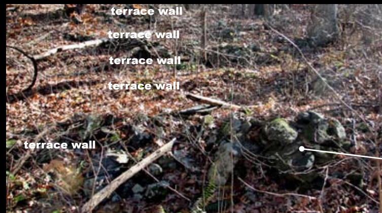
Series of crudely stacked stone terrace retaining walls
